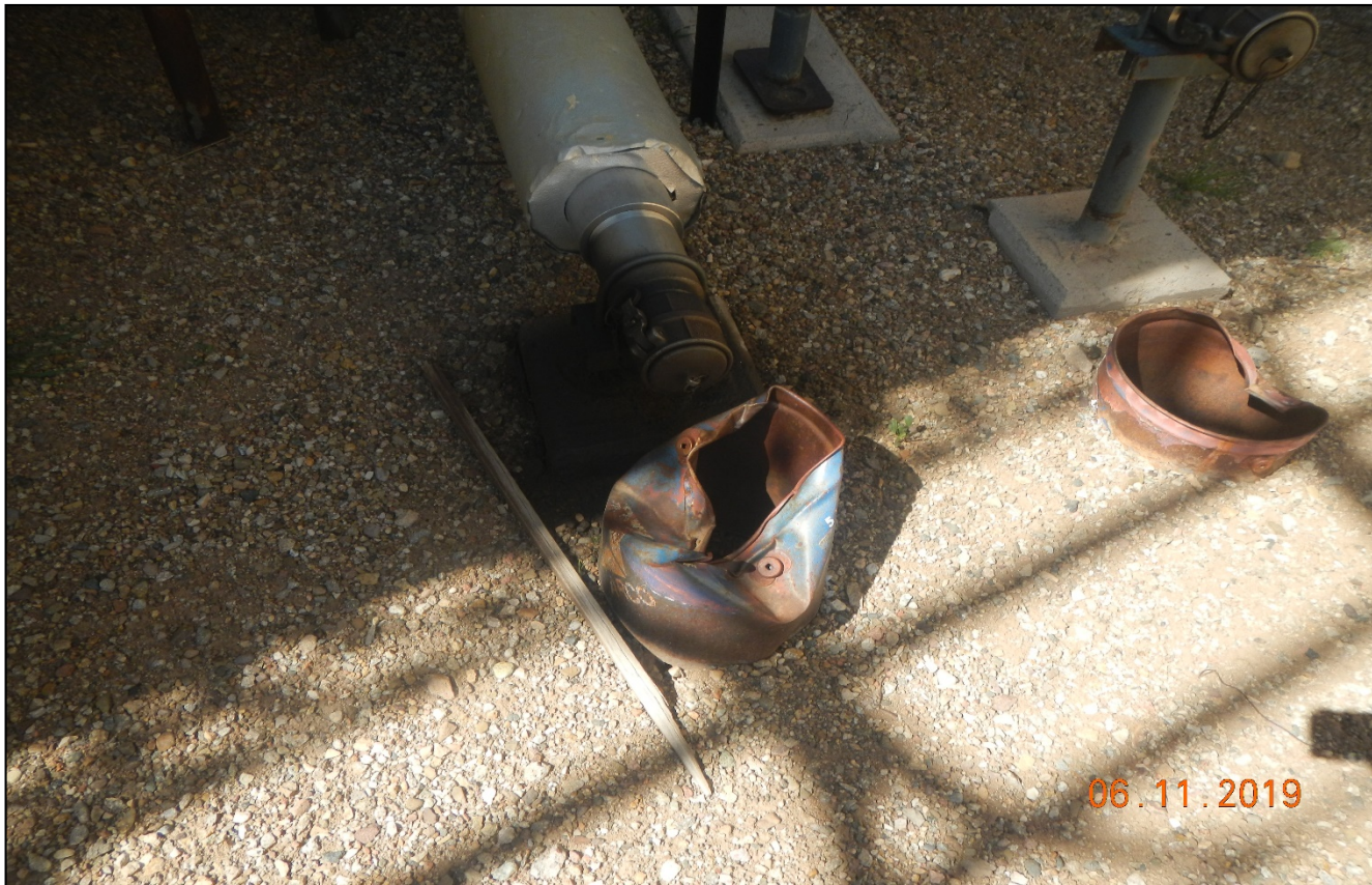
Photo 6. There is a bent bucket for secondary containment at the discharge point of the tank.
