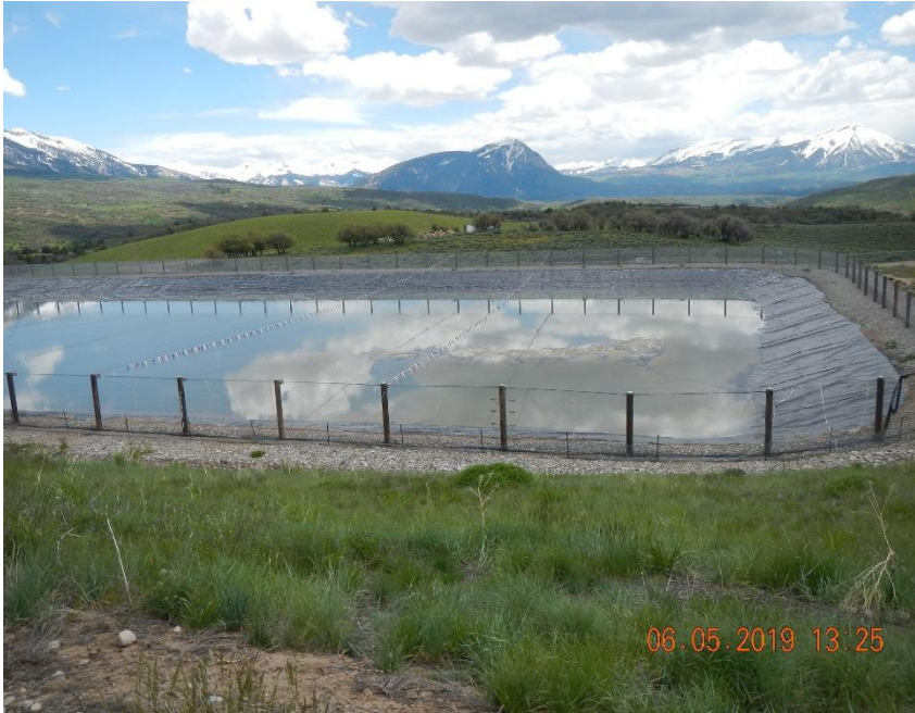
View of southern pit liner exposed.
