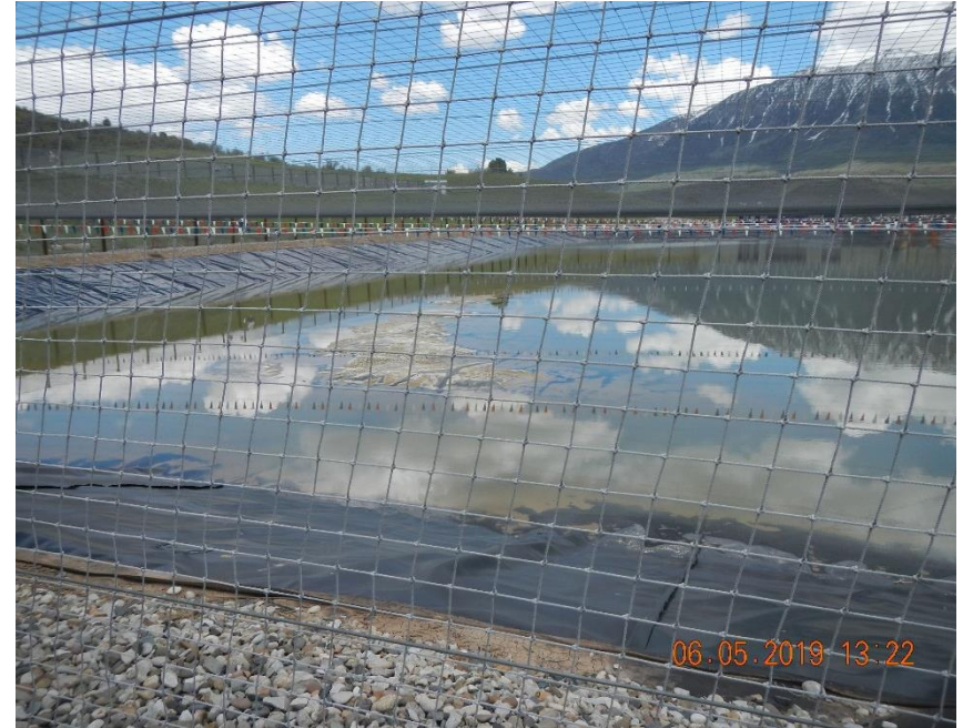
Bubbled up portion of liner in southern pit.
