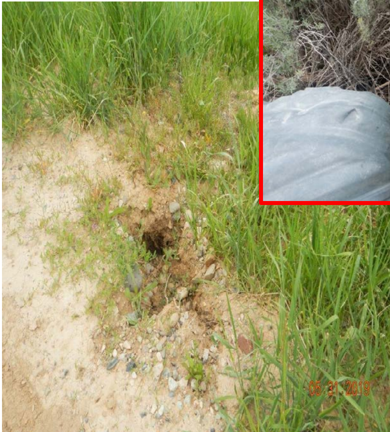
Photo#4: Subsidence at Culvert area.
