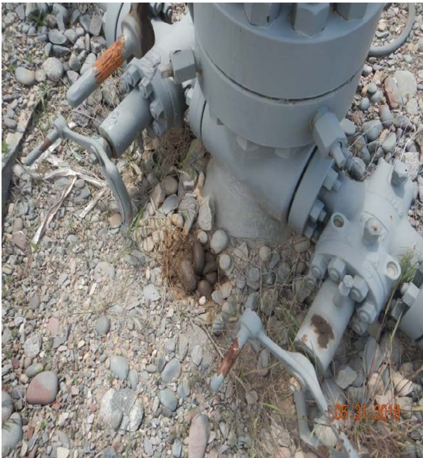
Photo#2: Staining at Wellhead.
