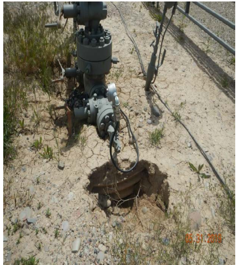
Photo#3: Subsidence at Wellhead.
