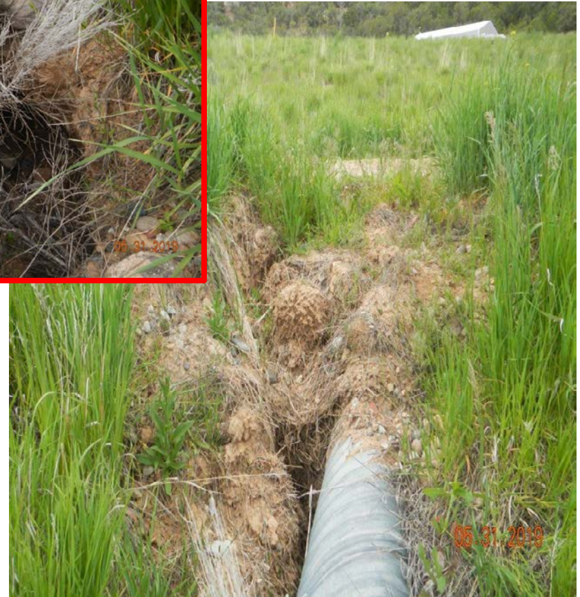
Photo#5: Subsidence at Culvert area.
