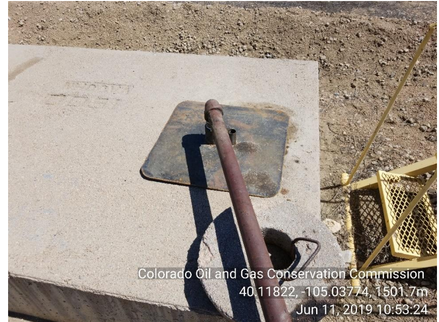
Photo 6 Produced water tank plate installed of opening
