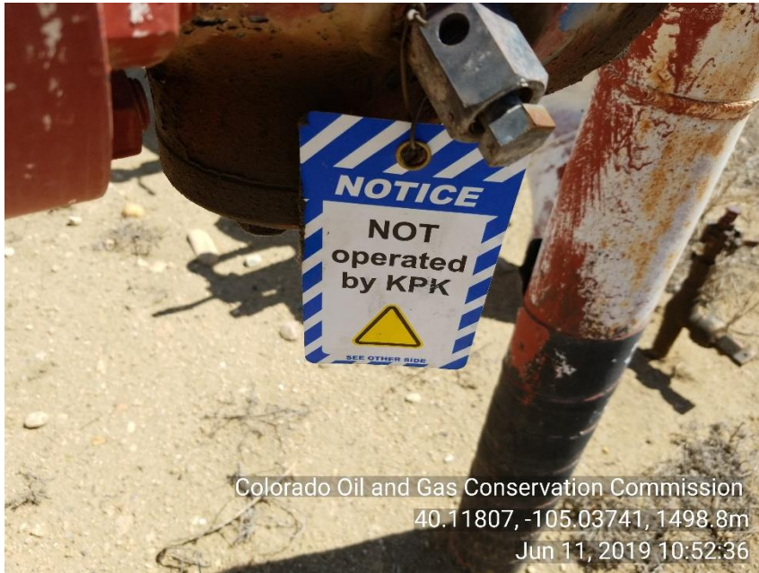
Photo 3 Unused flow lines have been marked
