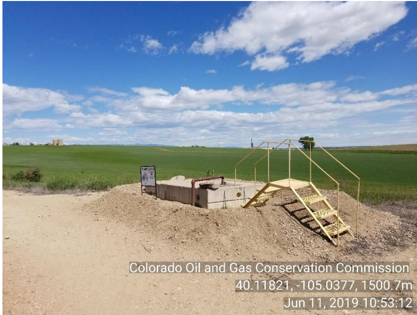
Photo 5 produced water tank berms have been repaired
