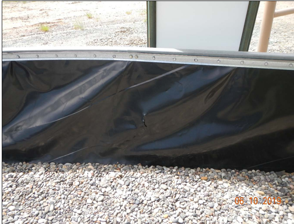
Photo #6 Holes in Tank liner.
