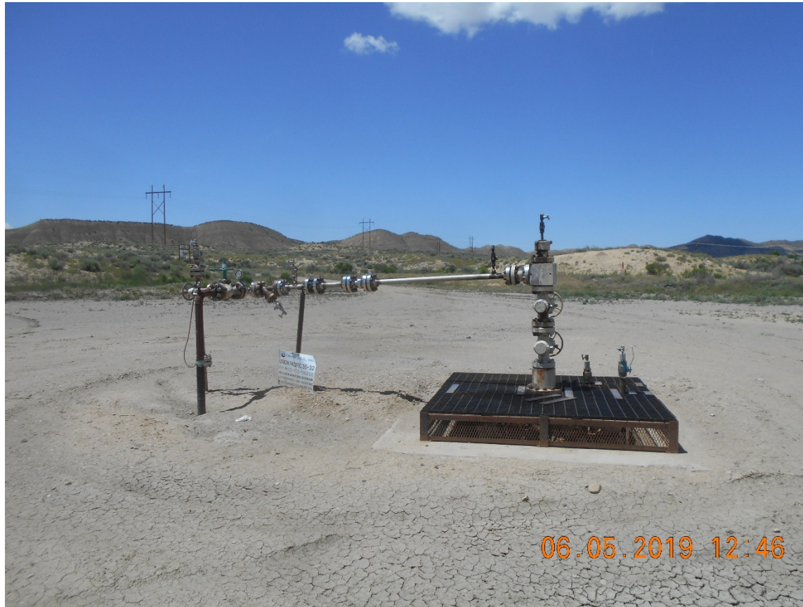
Injection wellhead
