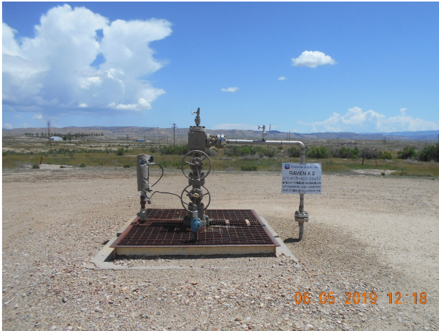
Injection wellhead
