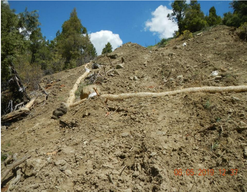
Wattles along south and west edges of stockpiled material.
