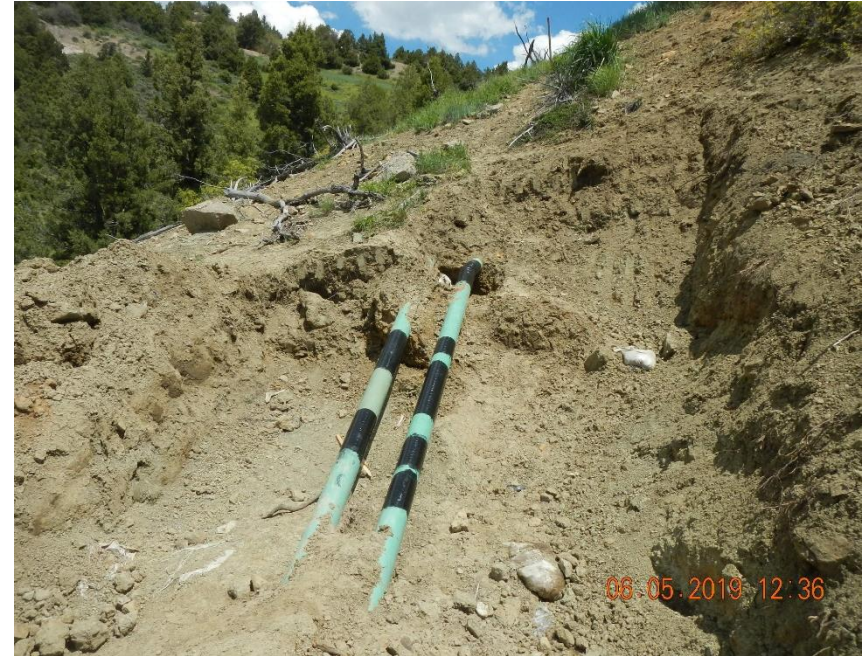
View uphill of excavated area. Produced water gathering line is on the left in this photo.
