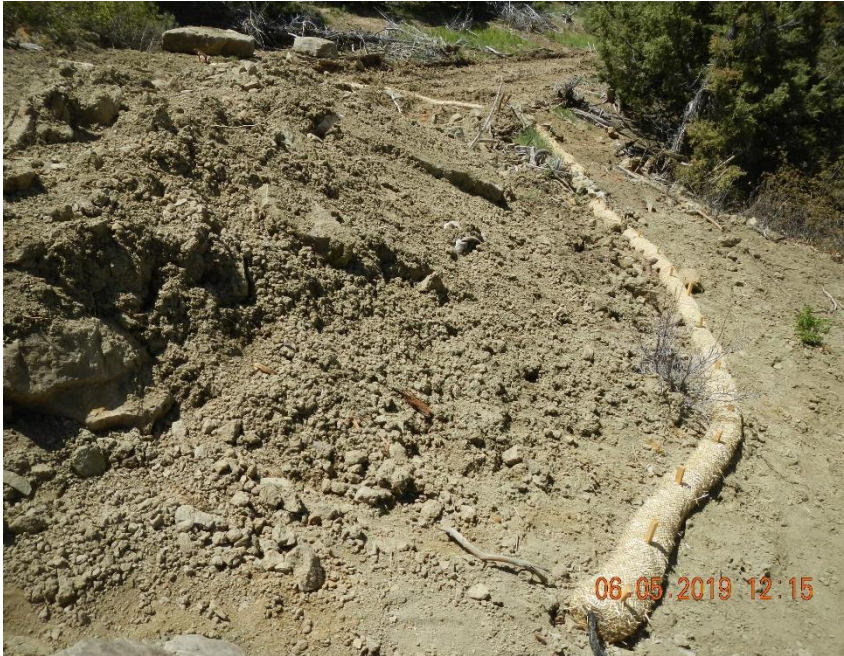
Soil stockpile from excavation of gathering lines.
