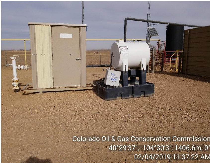
Photo 3 – Old Methanol Tank/Pump from previous inspection Doc ID 679600308
