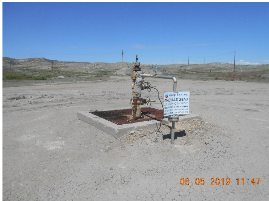
Injection wellhead
