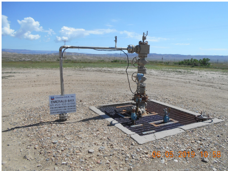
Injection wellhead
