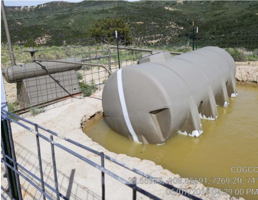
Photo 9. Blowdown tank floating in secondary containment.
