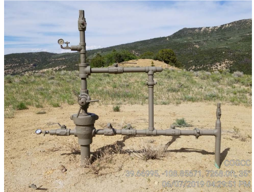
Photo 10. Wellhead without sign.
