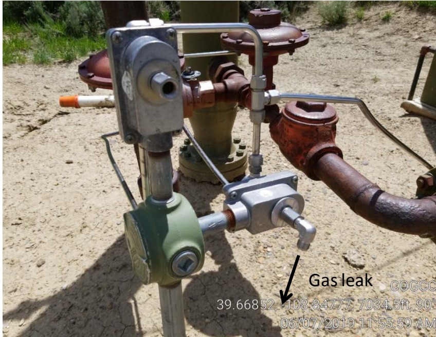
Photo 2. Gas leak at meter building.
