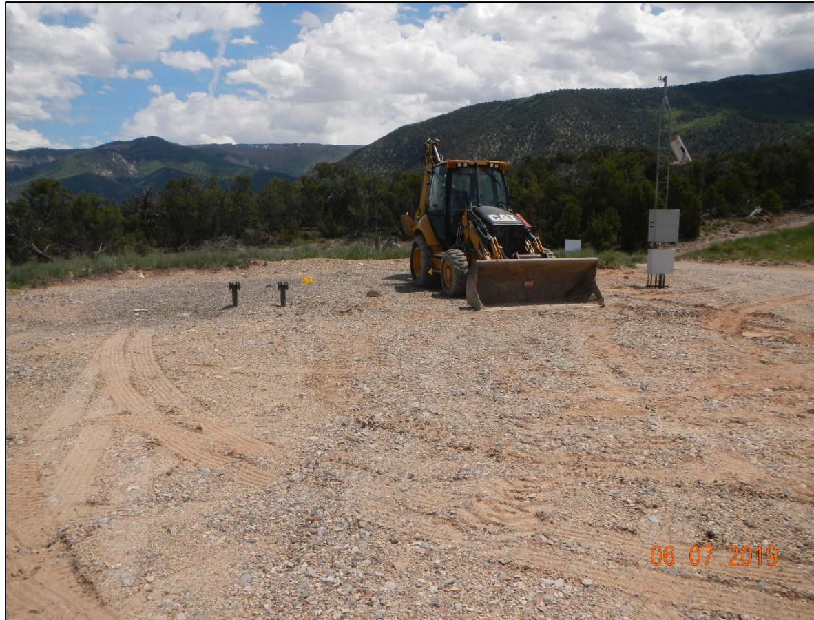
Photo #4 Photo of site location where production equipment has been removed. Risers are not locked out tagged out
