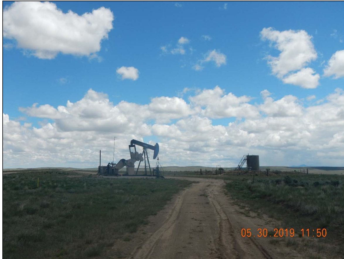
Photo 1. Overview of location taken facing north.
