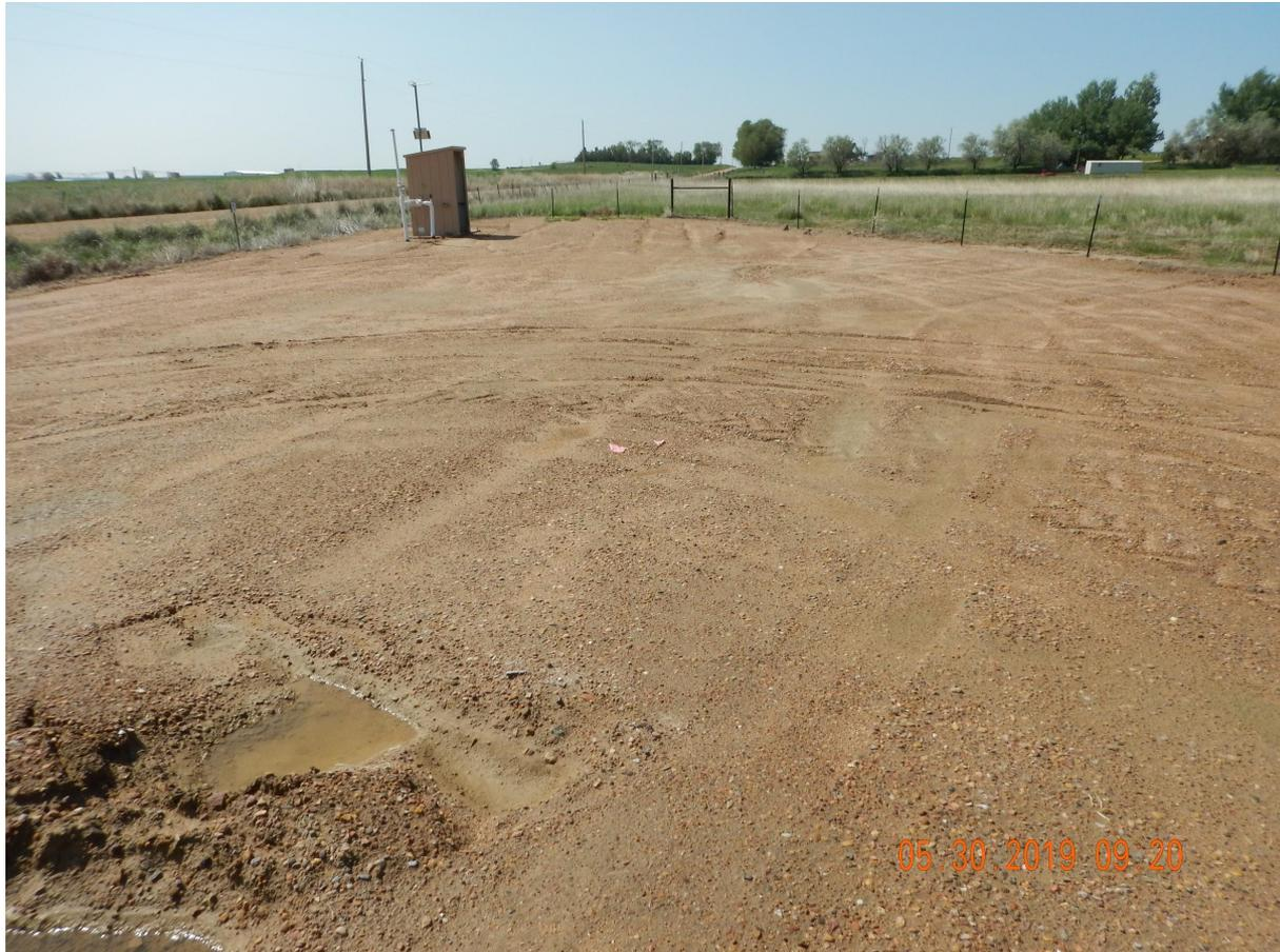
**Photo 1.** Photo taken from the southern tank battery, facing South. Operator indicated this southern tank battery was decommissioned on 2/13/2019. Photo illustrates it has been over 3 months and not all equipment has been removed from location. Per Rule 1004, Operator shall make every reasonable effort to perform final reclamation before the next local growing season.
