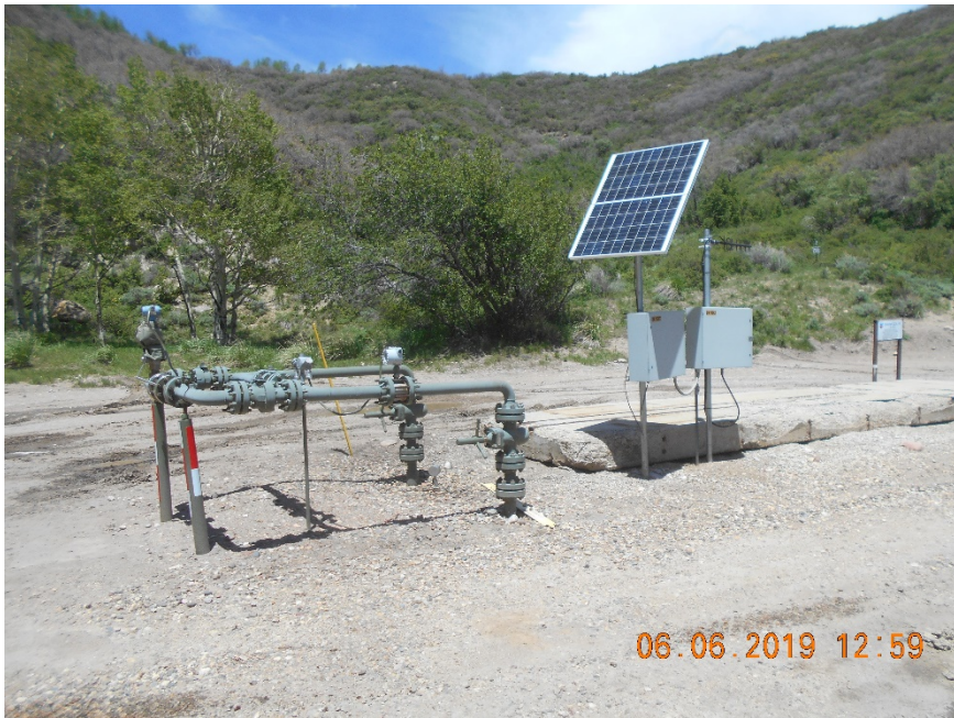
Injection wellhead
