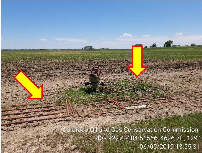
Photo 1 – Wellhead, Fence panel in despair.
