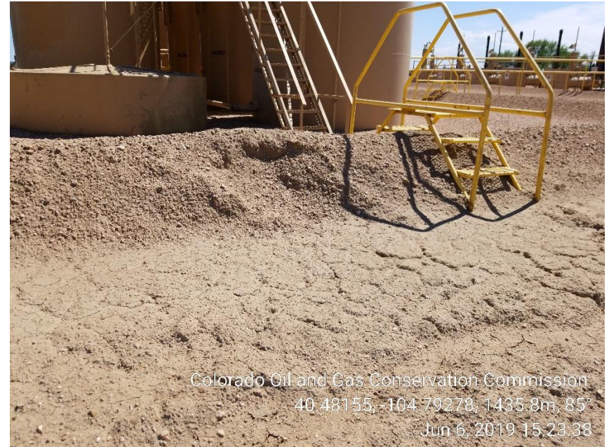
Photo 8: Berm in disrepair
