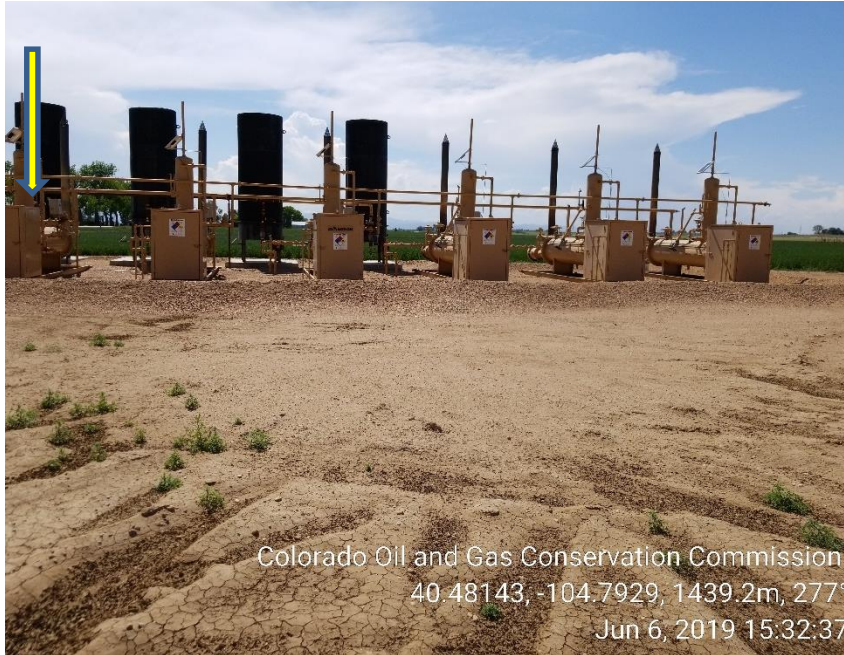
Photo 21: Separator that has stained soil
