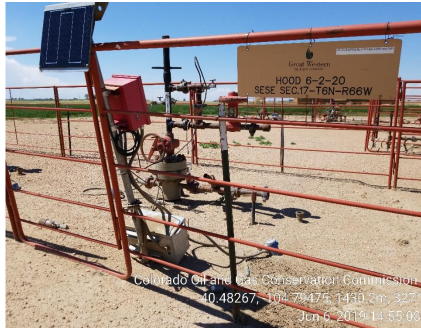
Photo 1: (TA) Wellhead; Unused equipment
