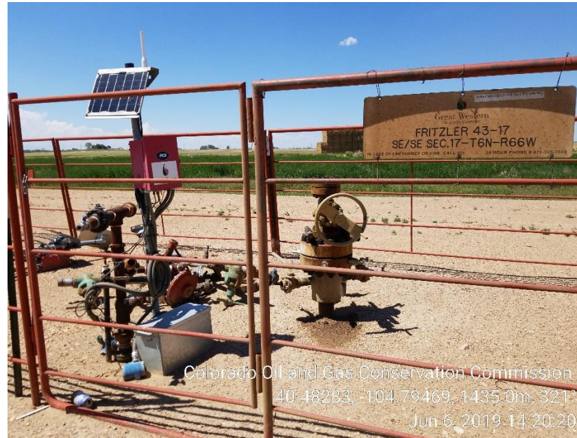
Photo 1: (TA) Wellhead; Unused equipment/stained soil
