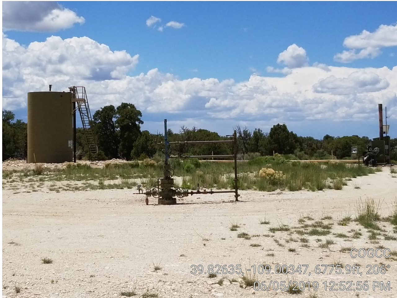
Photo 1. Location looking south.
