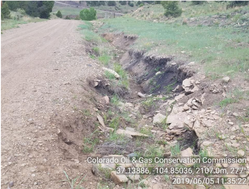
PHOTO 3: EROSION IN DRAINAGE DITCH ON MAIN LEASE ROAD APP. 75 YARDS WEST OF LOCATION ACCESS ROAD.
