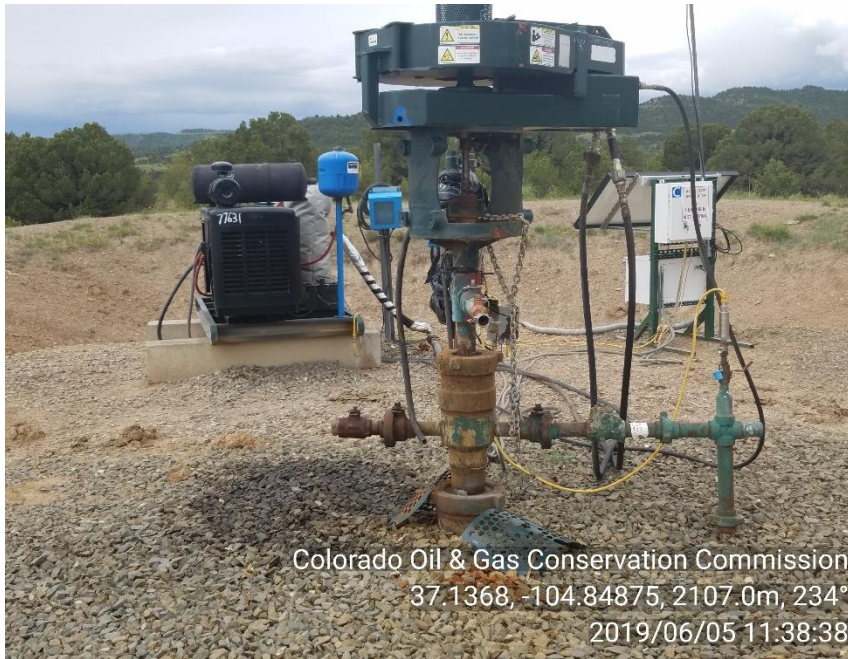
PHOTO 1: WELLHEAD/ APPROXIMATELY 3' BY 3' AREA OF IMPACTED SOIL NEAR WELLHEAD. Remove and dispose impacted material in approved manner, service and maintain equipment and self inspect to prevent recurrence of conditions per 1002.f(2) and 907" CA DATE 7/5/19
