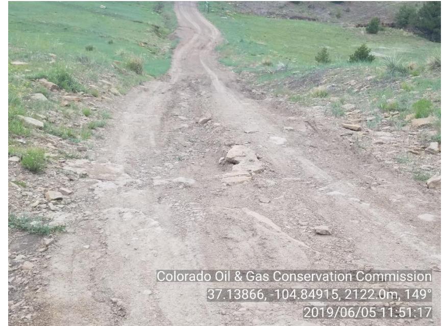
PHOTO 4: EROSION ON ACCESS ROAD JUST SOUTH OF ENTRANCE OF ACCESS ROAD. NO DRAINAGE DITCH OR BMP'S OBSERVED AT TIME OF INSPECTION. INSTALL PROPER DRAINAGE AND BMP'S IN ACCORDANCE WITH 1002 SERIES RULES. CA DATE 7/5/19
