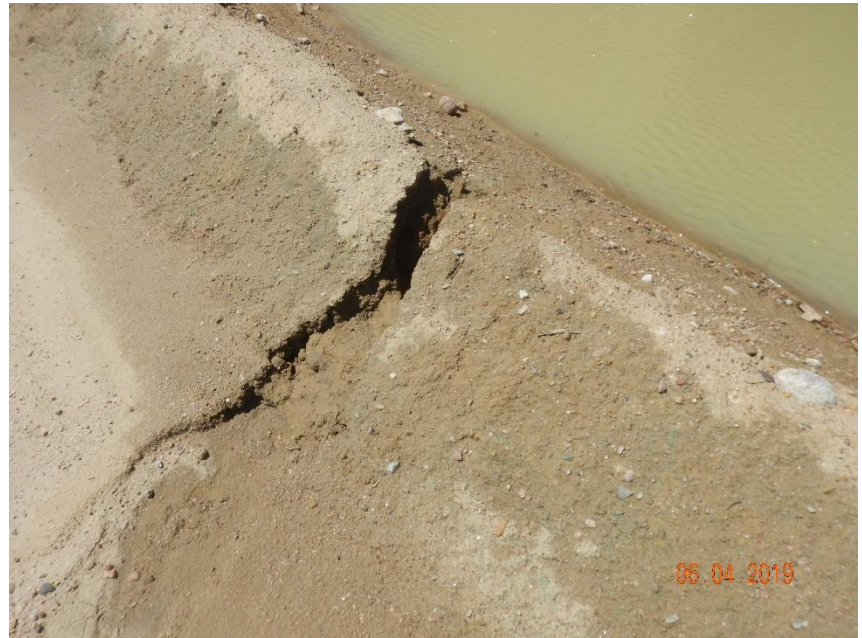
Photo 4: Continued from photo 3. Photo shows secondary containment is no longer in proper functioning condition in accordance with 906.d.(1)
