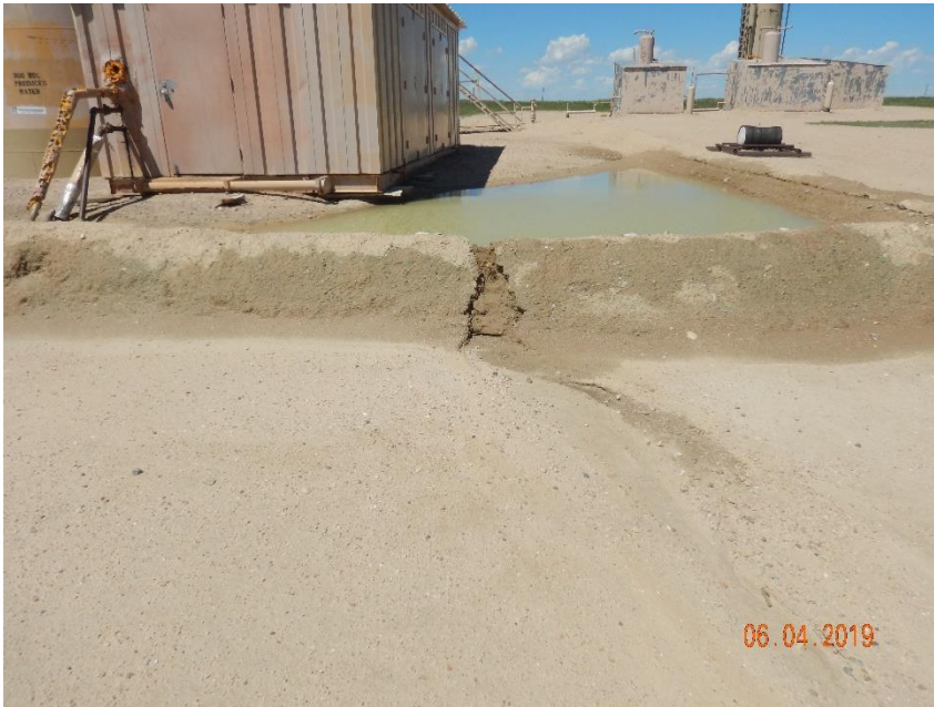
Photo 3: Photo taken from the southeast end of the location, facing west. Photo shows secondary containment is no longer in proper functioning condition in accordance with 906.d.(1)
