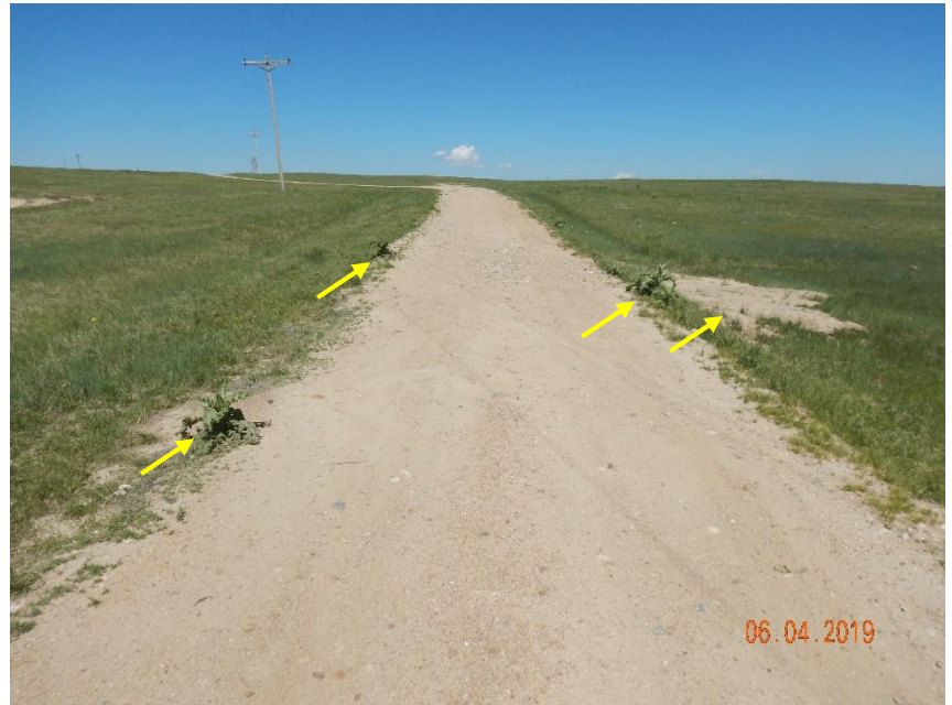
Photo 4: Photo taken from the main access road (approximately 40.650112°, -103.860646°), facing west. Photo shows Scotch thistle along access road. Photo also shows stormwater erosion degradation and sediment transport from the access road.
