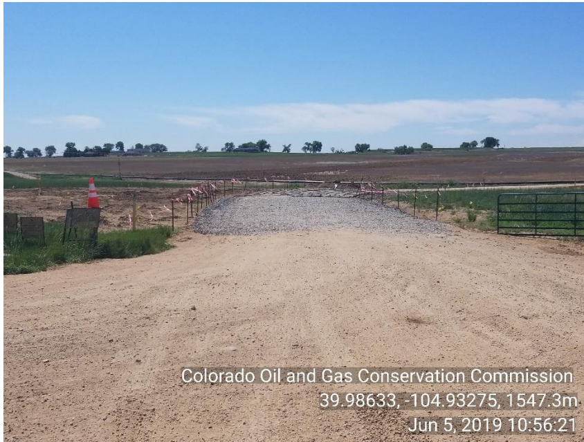
Photo 7 Tracking pad from HWY 7 into location
