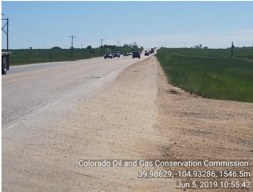
Photo 5 sediment being carried onto HWY 7
