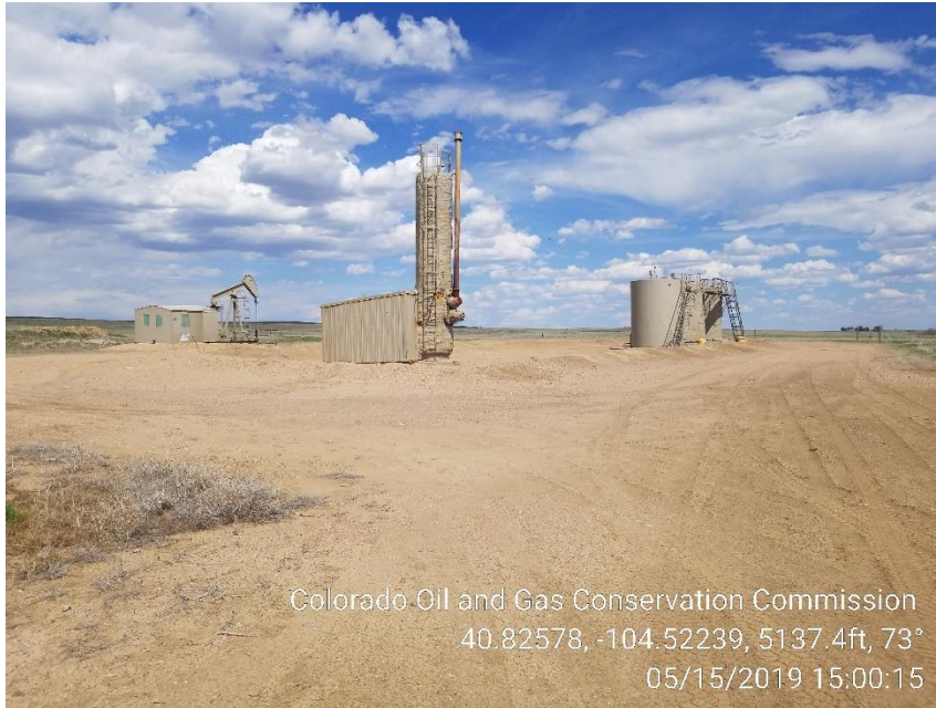
Photo 3 – Tank Battery
