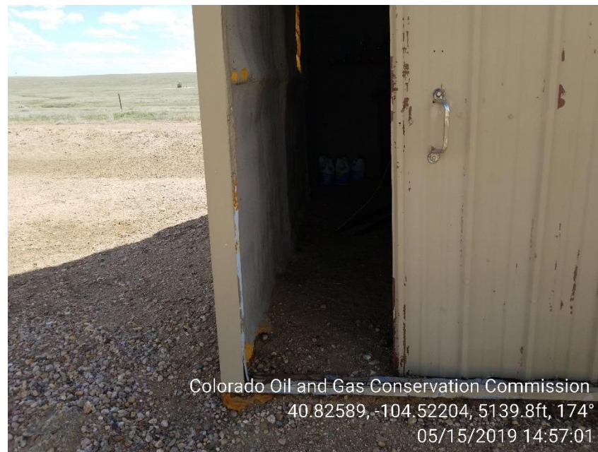
Photo 6 – Trash has been removed
