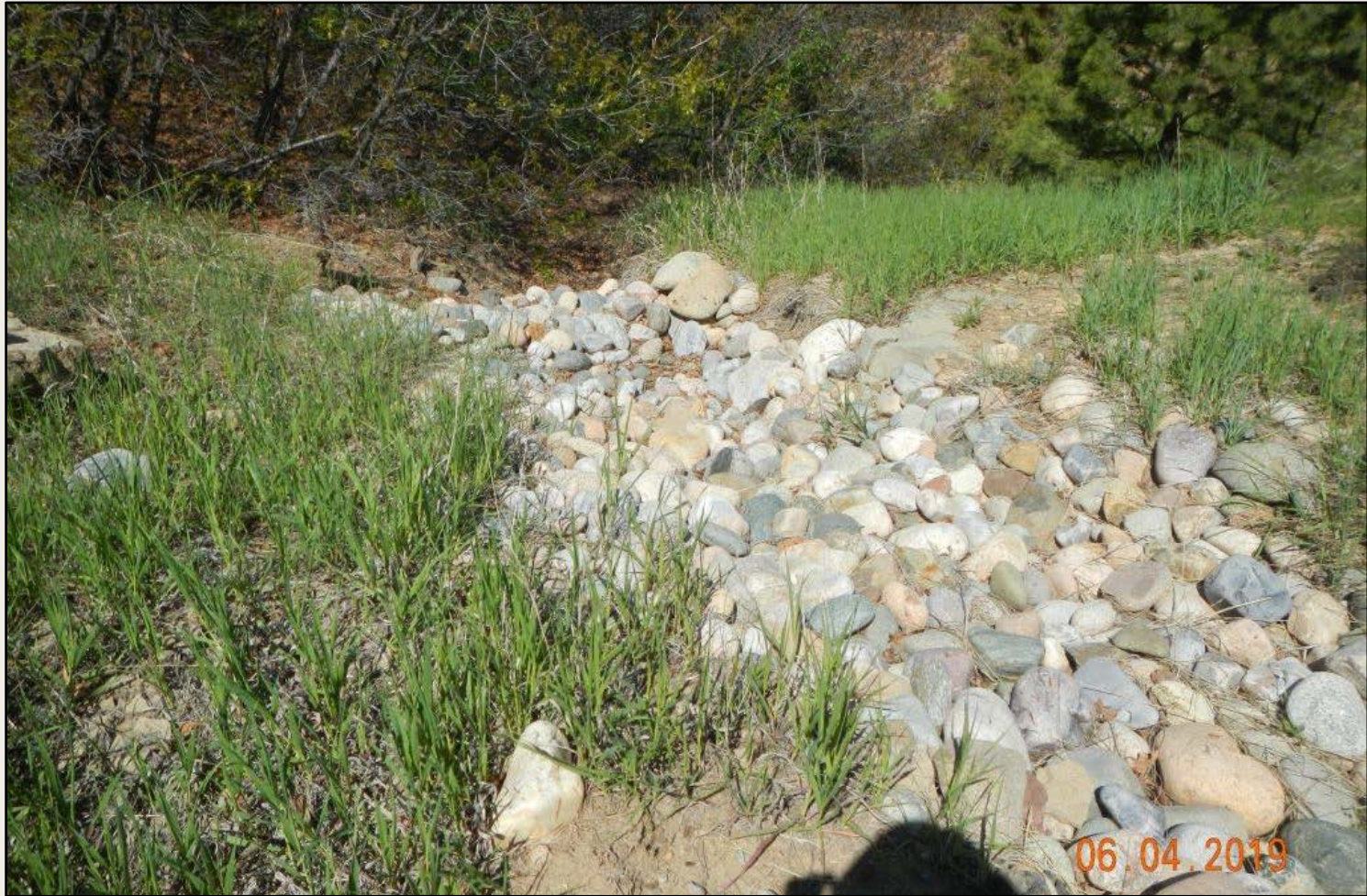
Photo 2. View of cobble run-down within the southwestern project area.
