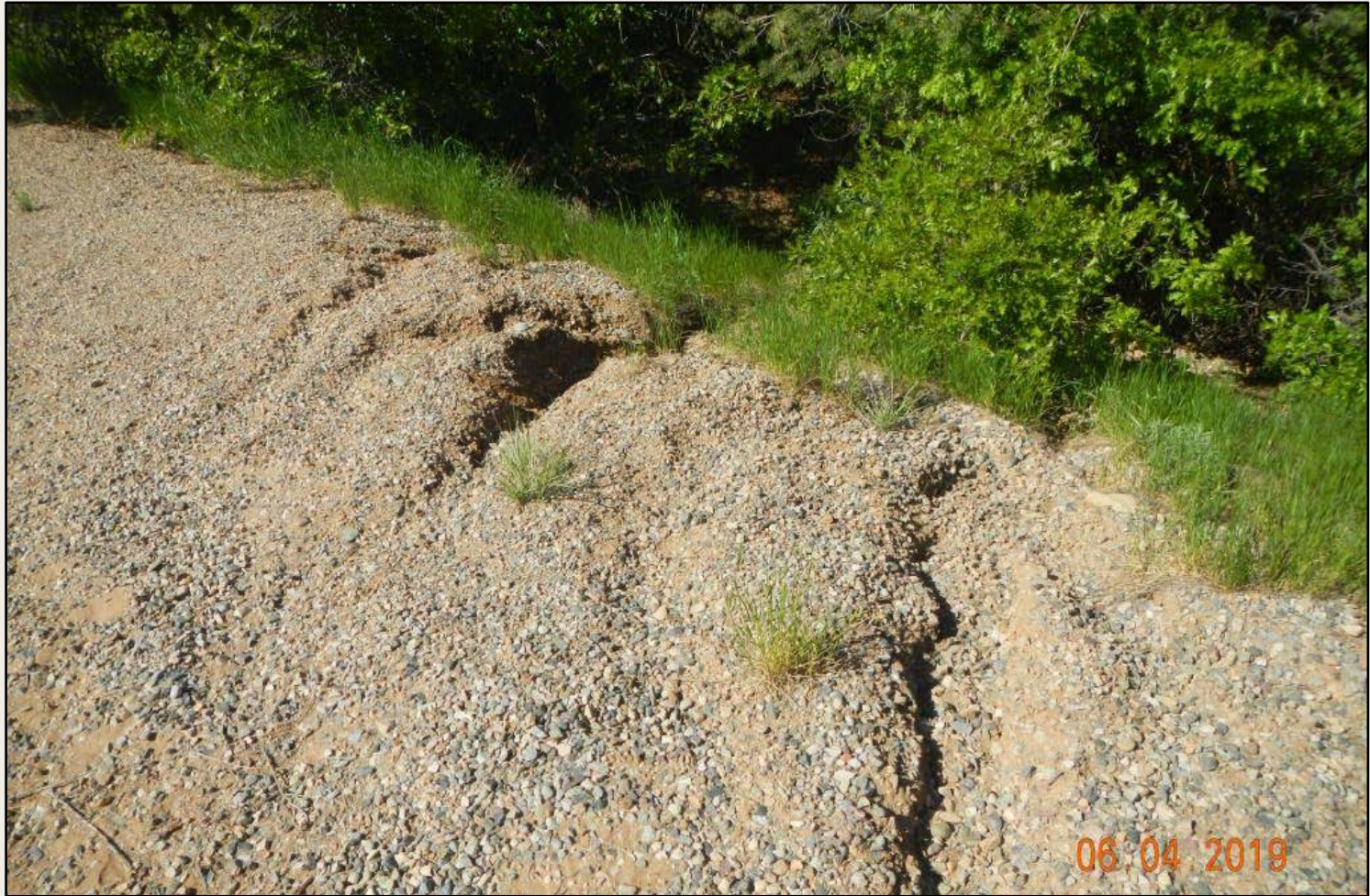
Photo 4. View of erosional rilling, up to 10 inches deep within the access road.
