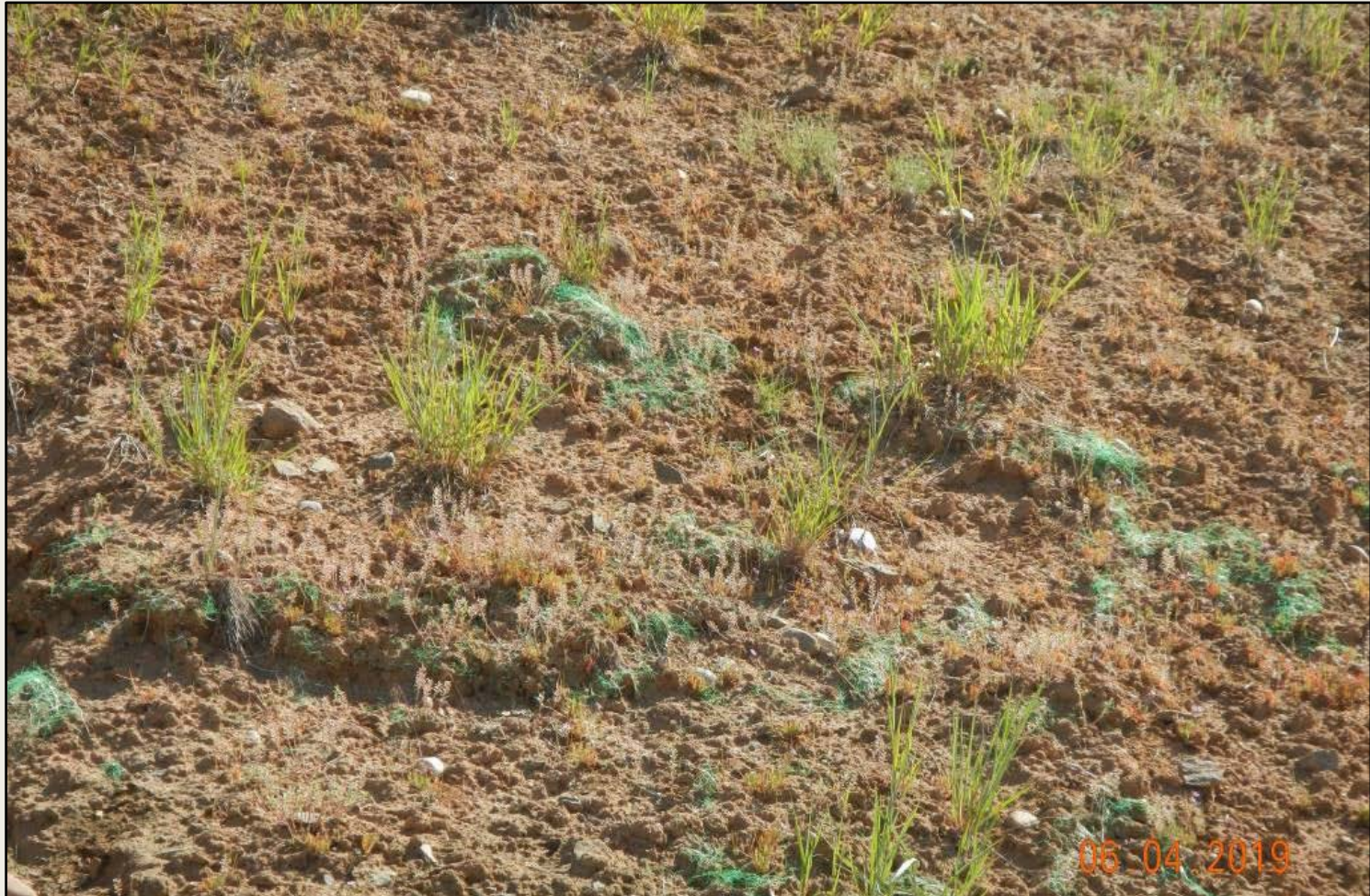
Photo 3. View of green plastic netting debris within the eastern cut-slope.
