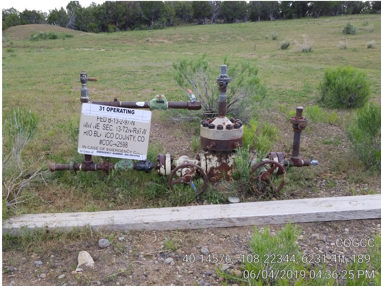
Photo 1. Inspection looking south.
