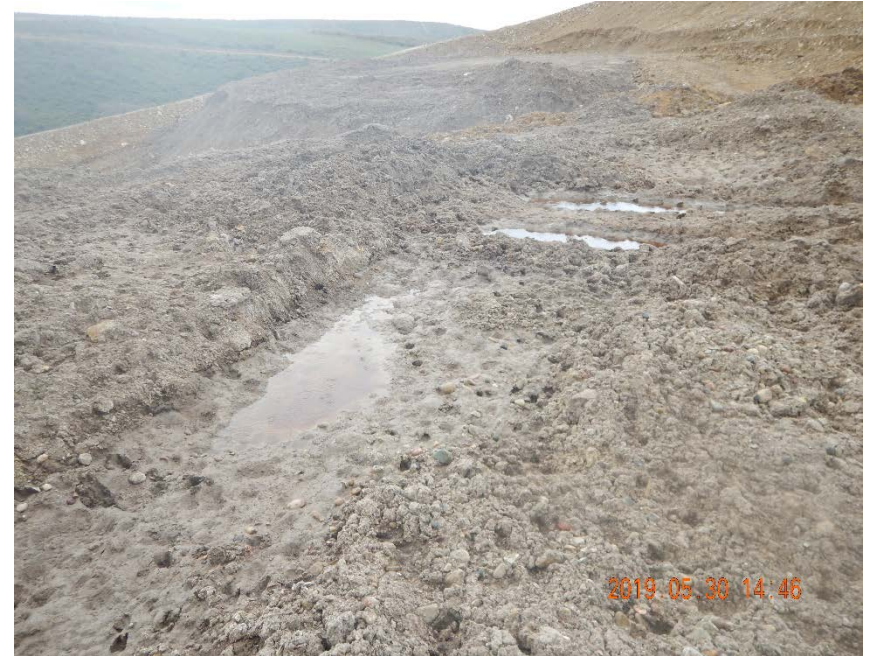
Photo #4 – Stormwater accumulation on top of cuttings pile. Note: it was raining during field inspection.
