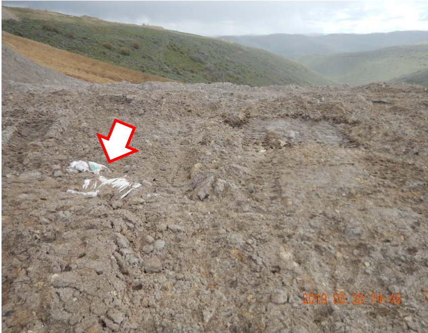
Photo #5 – Stormwater accumulation and trash on top of west cuttings pile.
