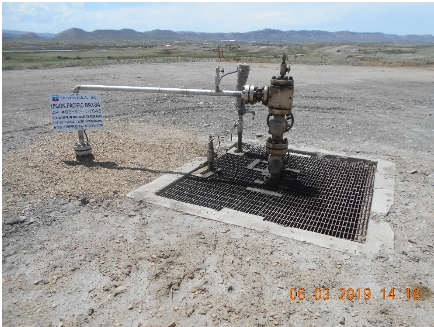
Injection wellhead
