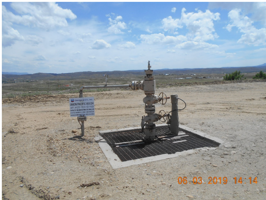
Injection wellhead
