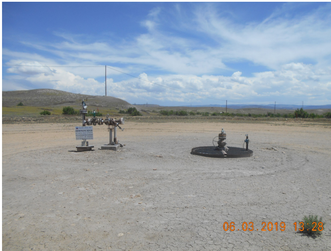
Injection wellhead
