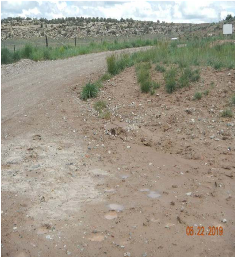
Photo#4: Run-on is occurring at access road entry
