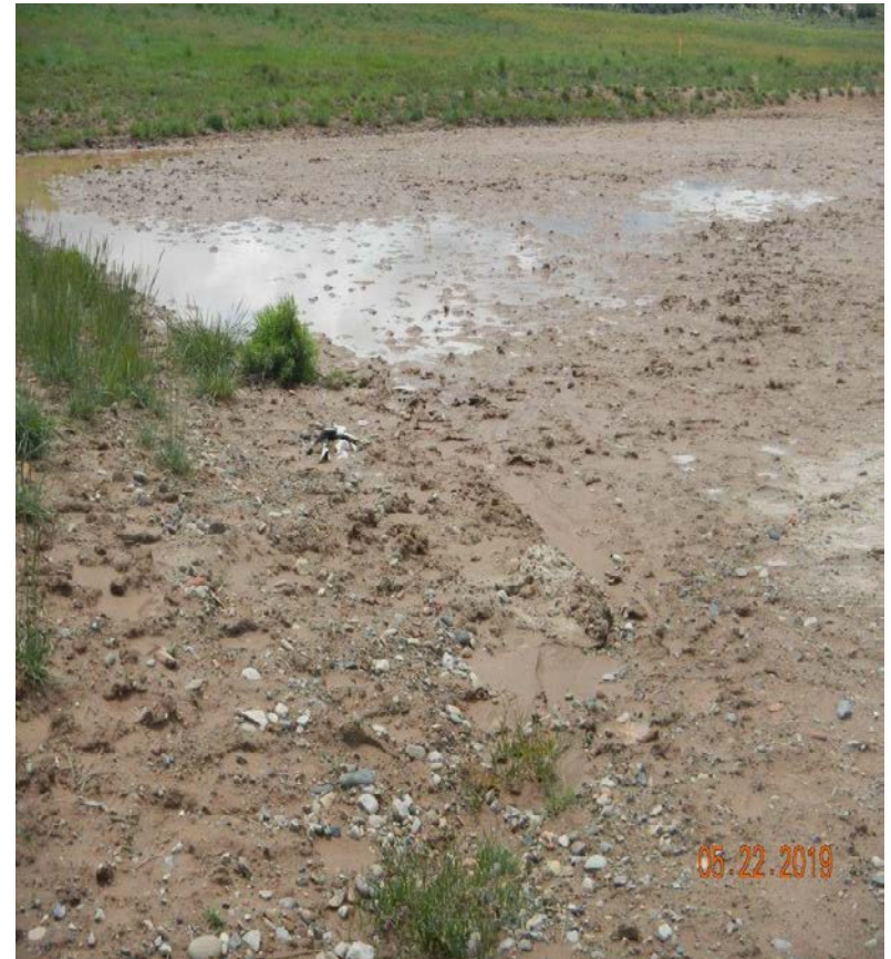
Photo#5: Run-on is occurring at access road entry.
