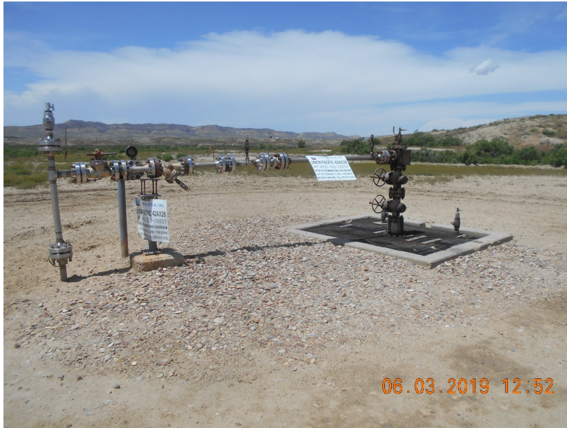
Injection wellhead
