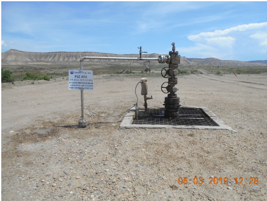
Injection wellhead
