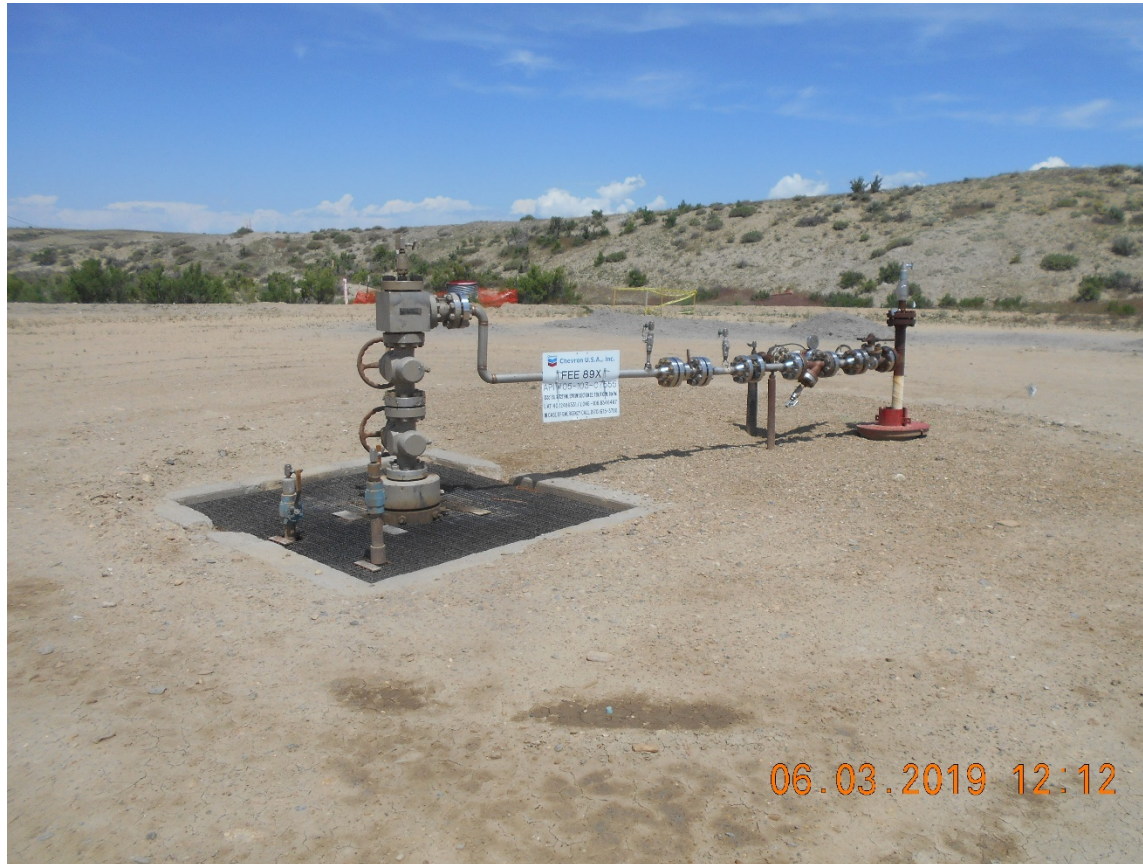
Injection wellhead
