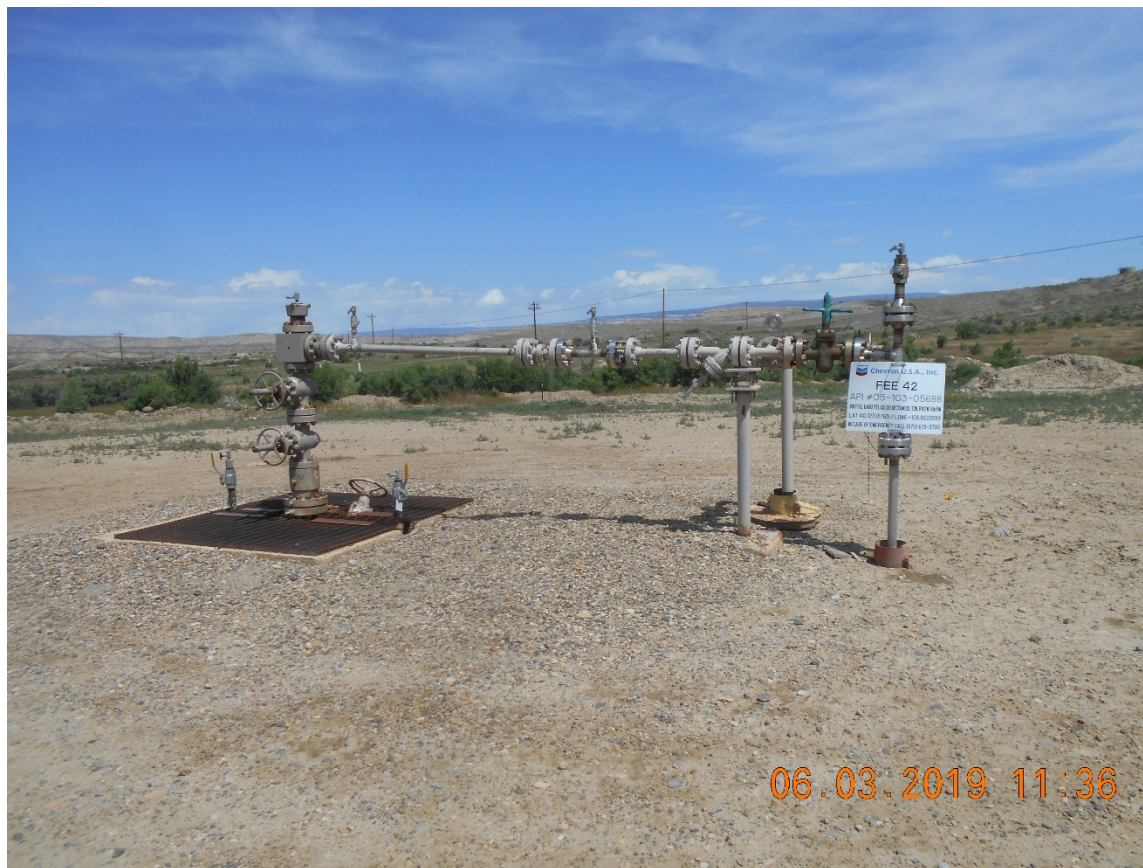
Injection wellhead – Temporarily Abandoned
