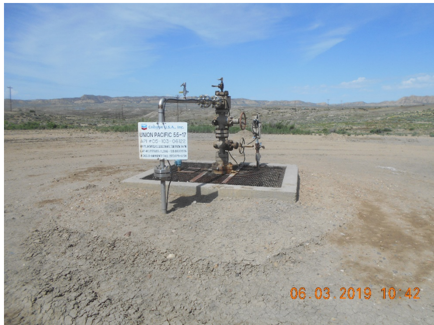
Injection wellhead
