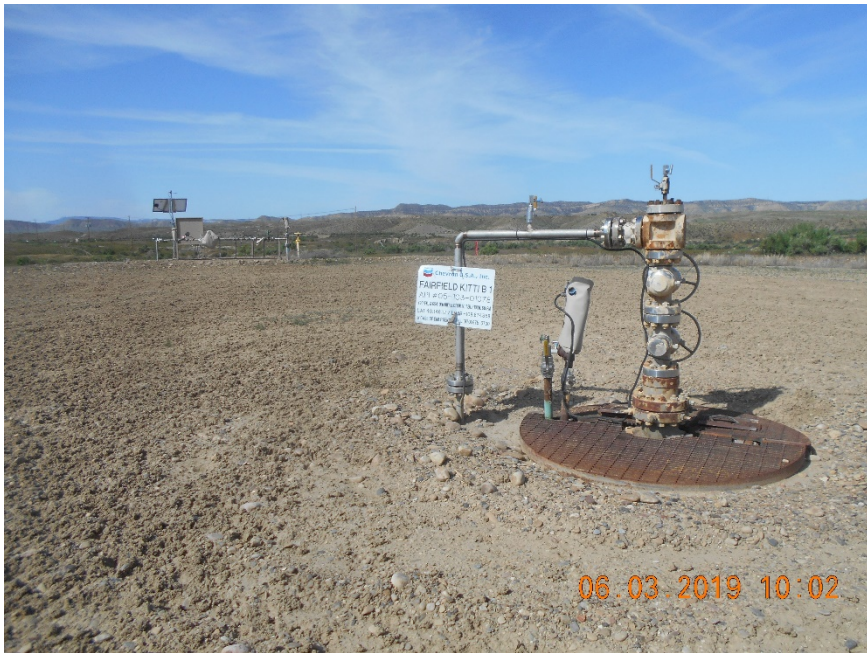
Injection wellhead
