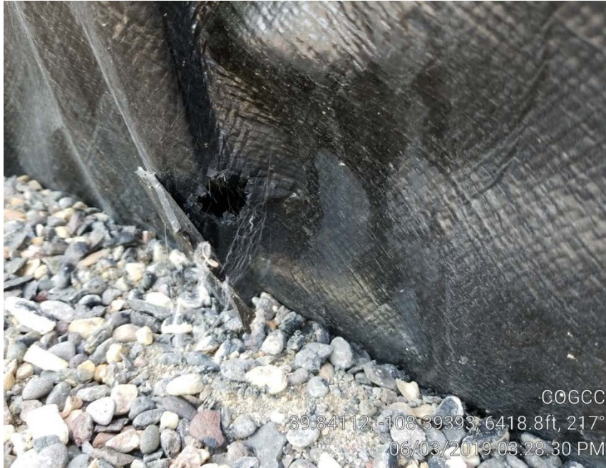
Photo 2. Liner repair inadequate.
