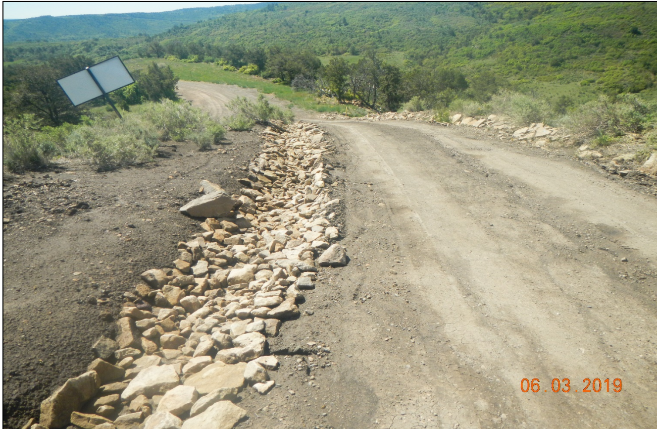
Photo 10. Rip/rap was added to control erosion.
