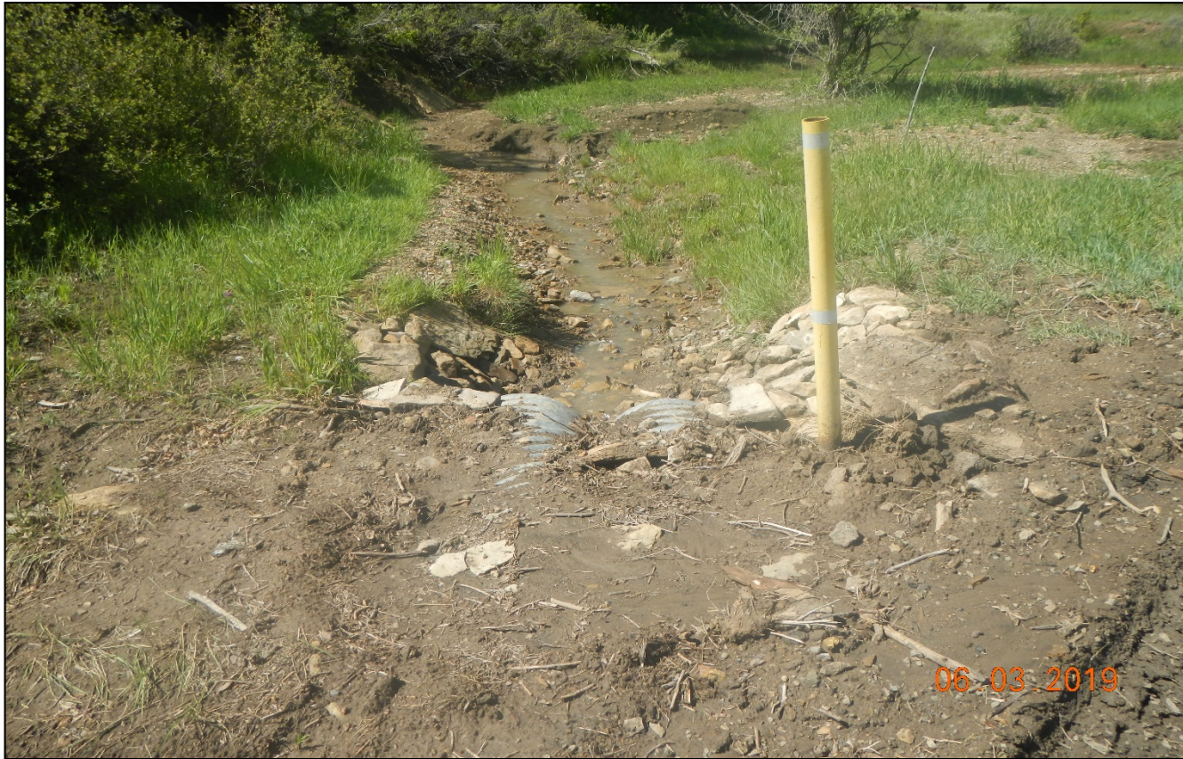
Photo 3. The culvert has been cleaned out and repaired.
