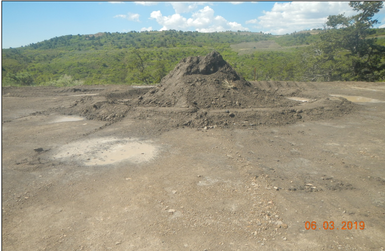
Photo 9. Berm was added around soil pile.
