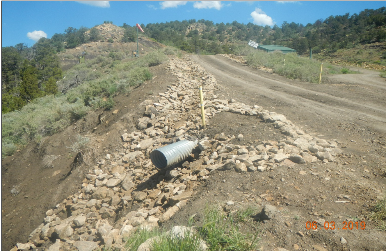
Photo 6. Additional rip/rap has been added to the outlet of the culvert.
