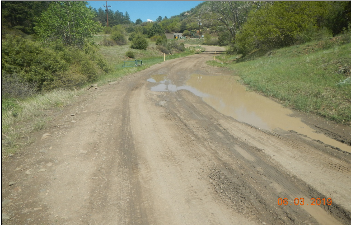
Photo 3. Stormwater is pooling onto the road and is not properly diverted.
