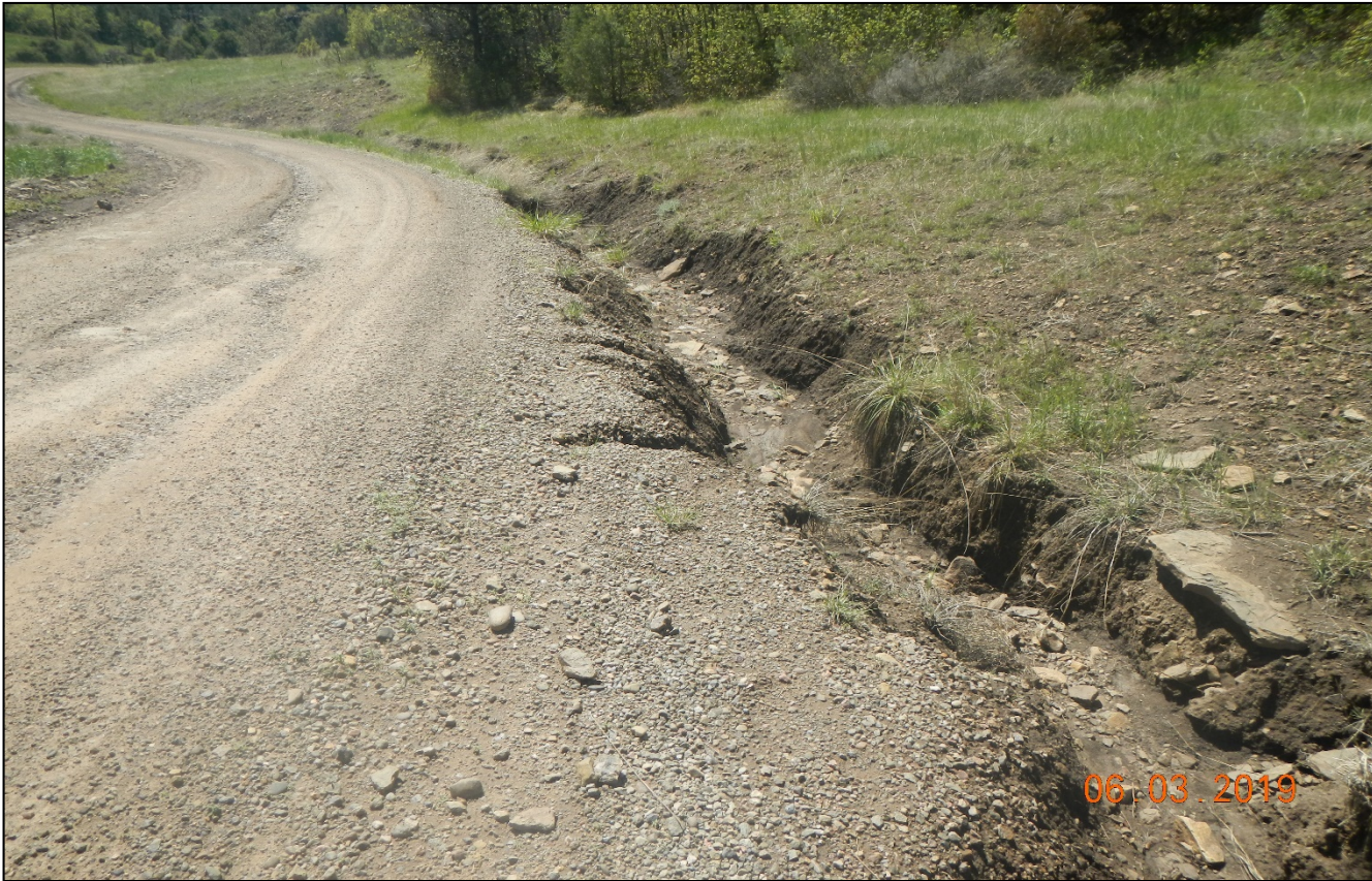
Photo 4. The erosion channel at the southeast side of the location has not been repaired.
