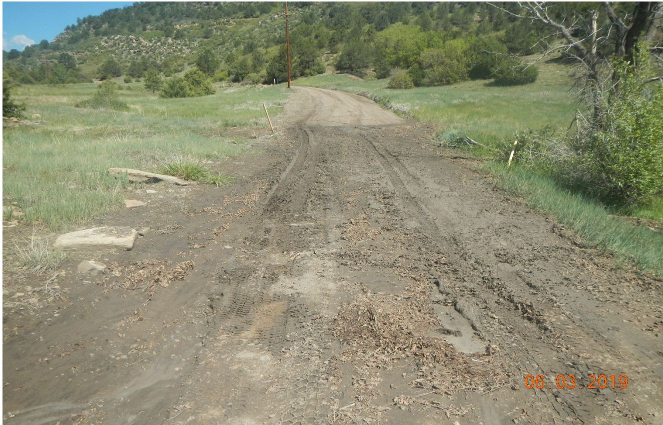
Photo 1. Facing northwest at mouth of the canyon. It appears stormwater has flowed across the road at this point causing damage.
