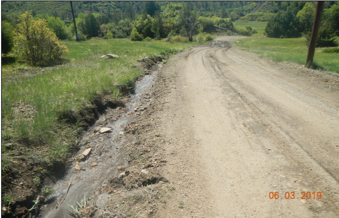
Photo 2. Facing back to the southeast. Erosion is occurring along the side of the road and no BMPs are installed (checkdamns).
