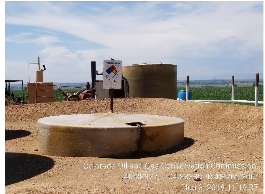
Photo 4: No BBLS listed on Produced Water Tank
