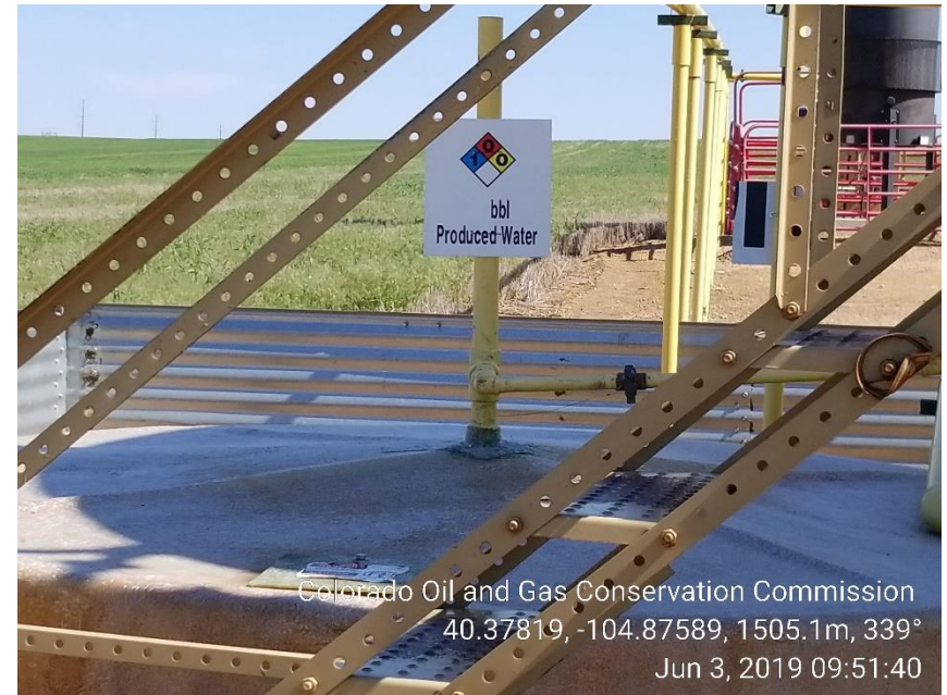
Photo 2: No BBLs listed on Produced Water Tank
