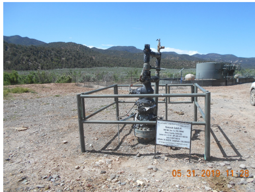
Injection Wellhead with fencing and sign
