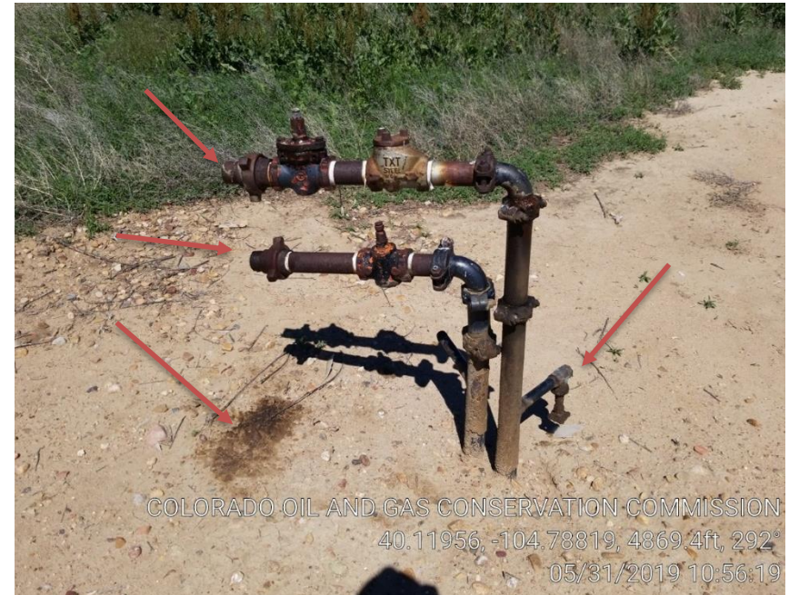
Pic 8 unused unmarked uncapped risers on location/stained soil
