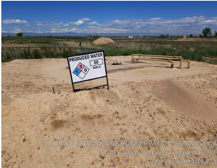
Pic 7 inadequate berms around water tank
