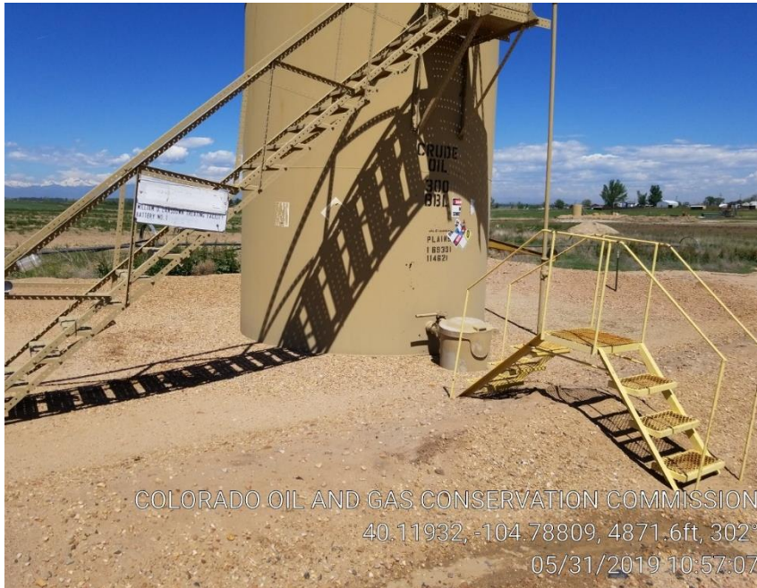
Pic 9 inadequate berms around oil tank, placards and sign is not legible
