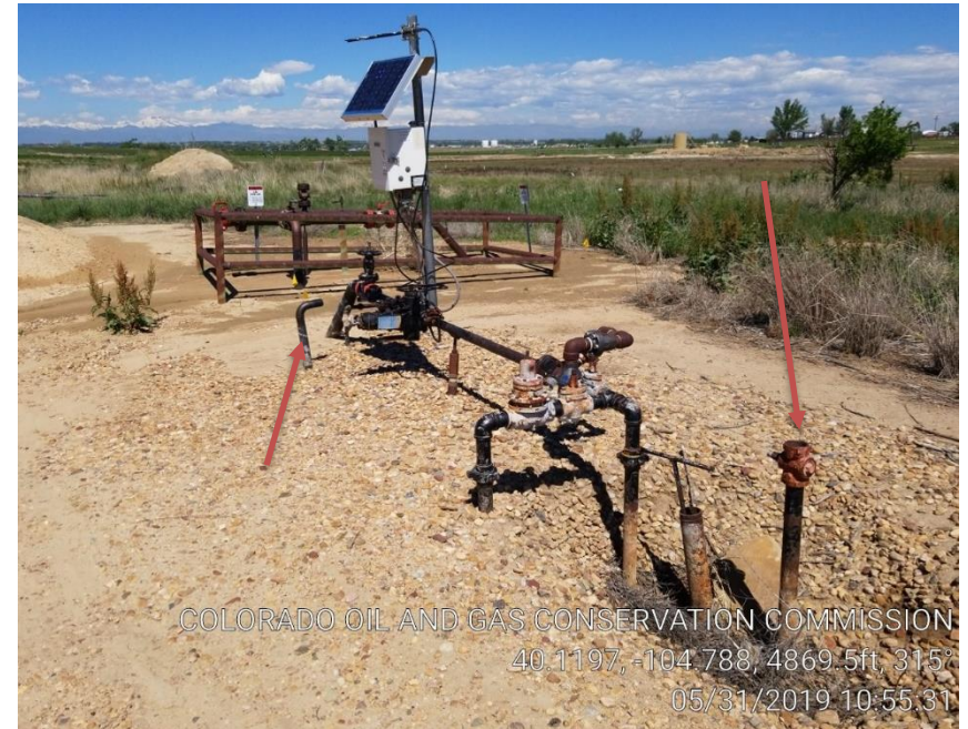
Pic 6 uncapped unmarked risers
