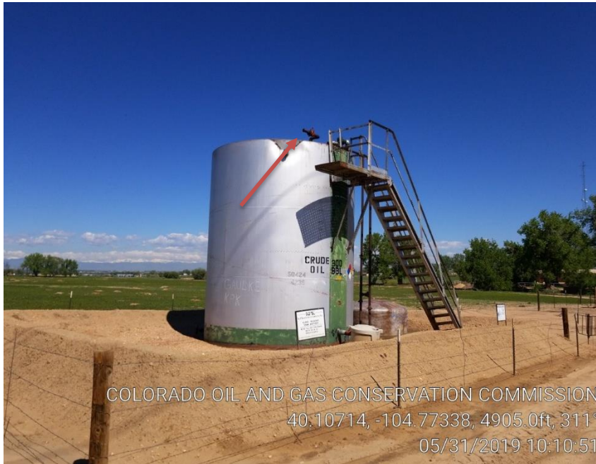
Pic 1 unpainted tank, uncapped lines on tank
