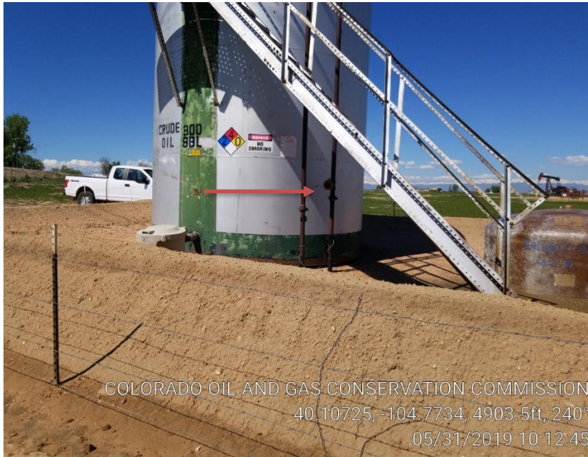
Pic 3 unpainted tank, uncapped line
