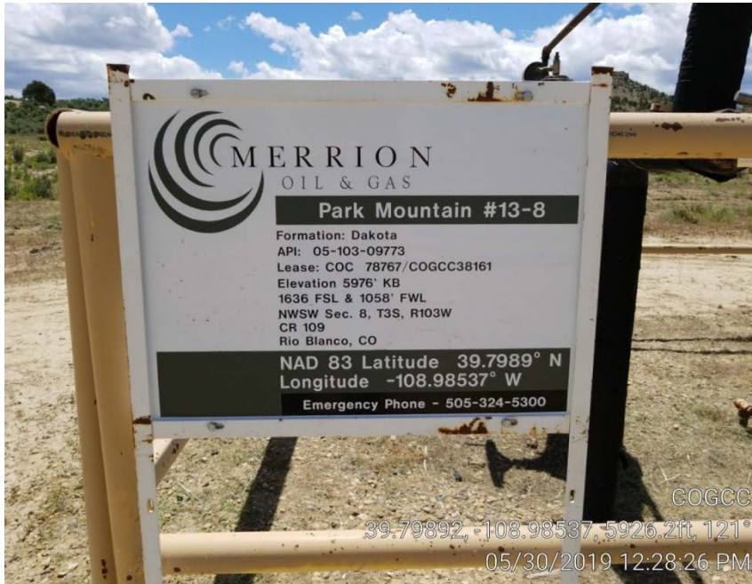
Photo 2. Sign missing Nearest Public Road & 911.
